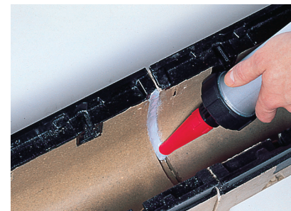
Sealant applied with caulk gun
