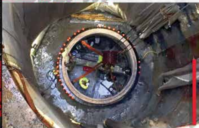
160 FEET DEEP (48.8 METER) UTILITY ACCESS 14 FEET (4.3 METER) DIAMETER PRECAST MANHOLE
