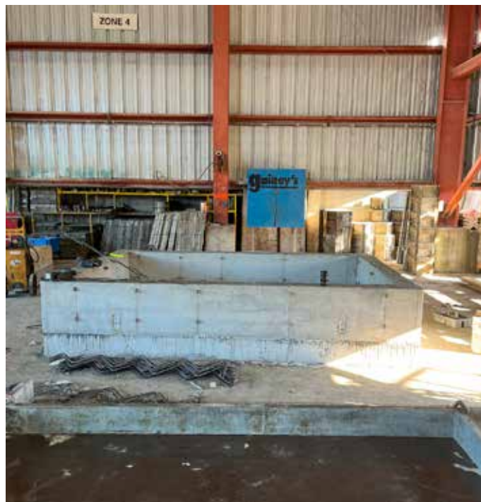
Gainey’s constructed a replacement for the damaged top and walls of the wet well vault plus two risers and a flat top section, in addition to a vault box and a PRV structure for the community of Lake Lure, North Carolina.
