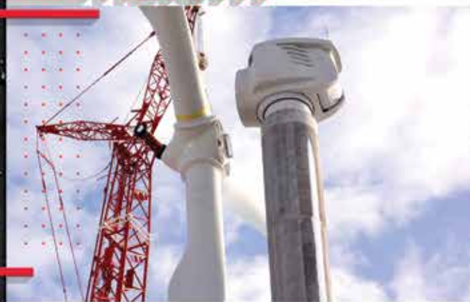
100 METER TALL (328 FEET) PRECAST WIND TURBINE TOWER
