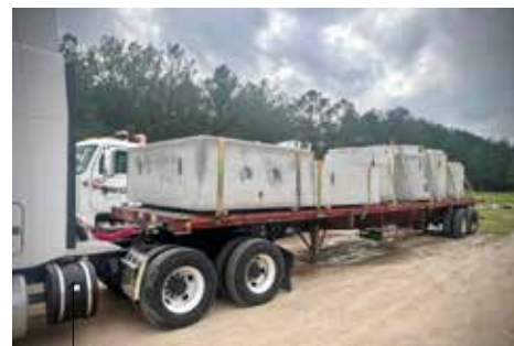
The custom precast pieces traveled more than 700 miles to be installed.
