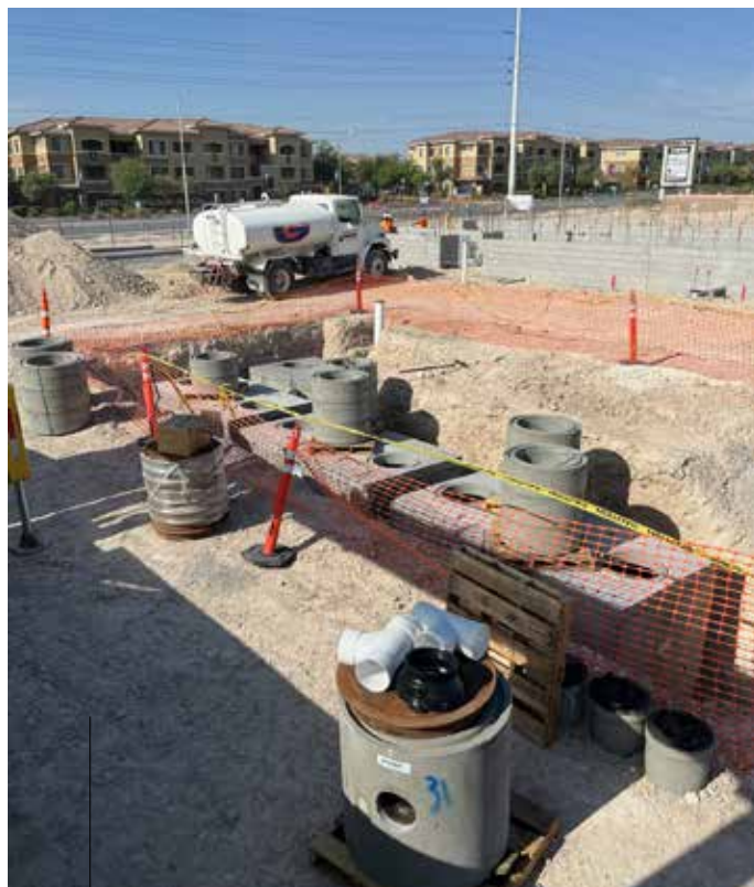
Precast is playing an important role in the construction of eco-friendly car washes in Las Vegas. The material's inherent strength and durability make it ideal for capturing and storing large volumes of water.
