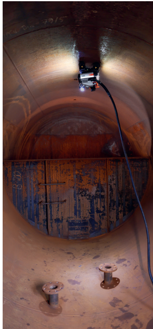
Working upside down? No problem for this robot!
