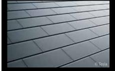
Tesla's Solar Roof technology uses photovoltaic tiles to cover entire roofs. Technically, they function like any other traditional solar panel. However, there is a major difference from an aesthetic point of view, as these tiles, quite similar to normal tiles, are the first to be actually integrated into the roof. Also, they are extremely durable and weather-resistant. Tesla guarantees them throughout the building's entire lifespan.
