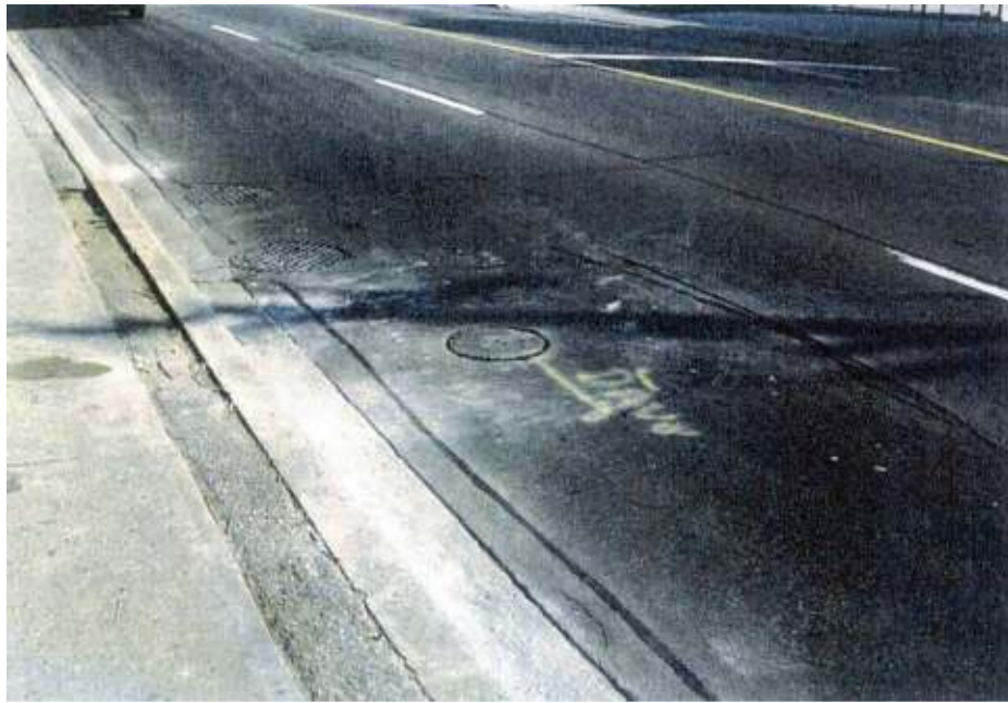
Figure 10 – View of reinstatement two weeks after installation
