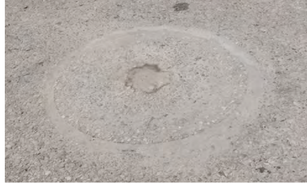
Figure 12: Reinstated 18-inch diameter core. Courtesy Utilicor Technologies Inc.
