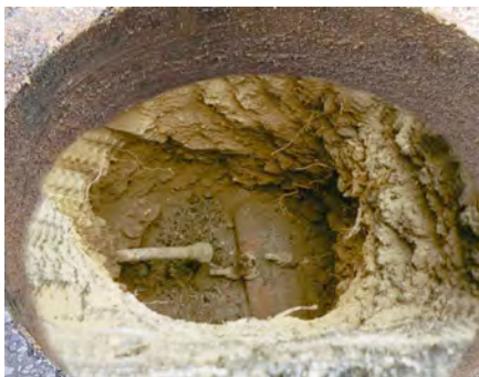
Figure 4: Excavated keyhole showing lateral and original 6-inch cast iron main. AwwaRF 2007
