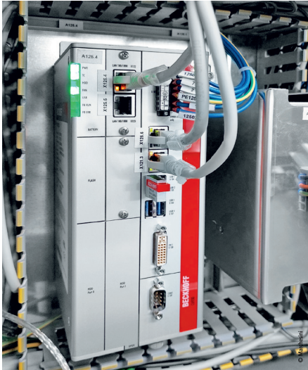
Marchesini uses a C6930 control cabinet industrial PC to automate the entire Compact-24 filling line.
