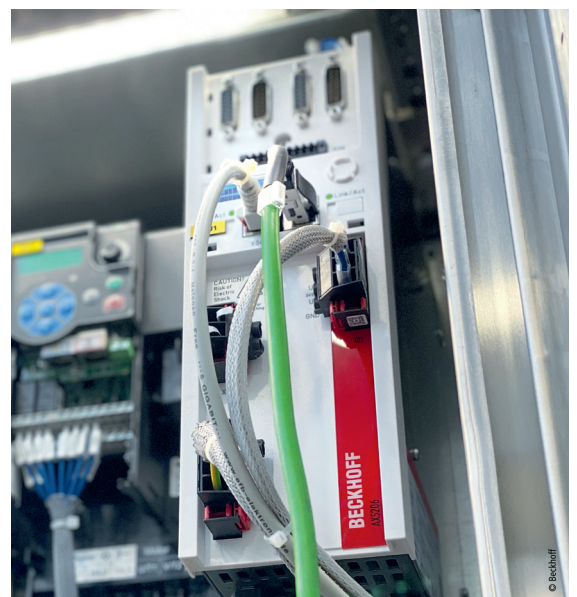
Fast control of the pressure pump – via the AX5000 servo drive and AM8000 servomotor – is crucial for precise filling.
