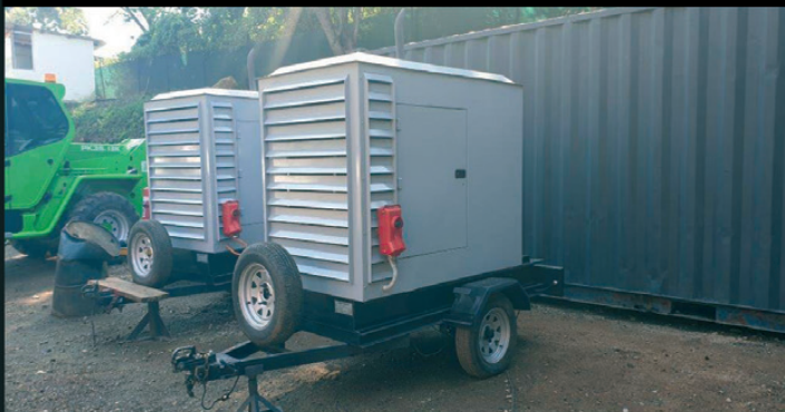
2 X 40KVA GENSETS WITH 3 PHASE POWER
