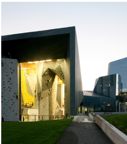
Salewa Headquarters, Bolzano/Italy (2007-2011)
