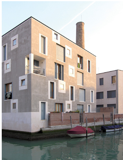
D Residential Building, Venezia/Italy (1997-2003)
