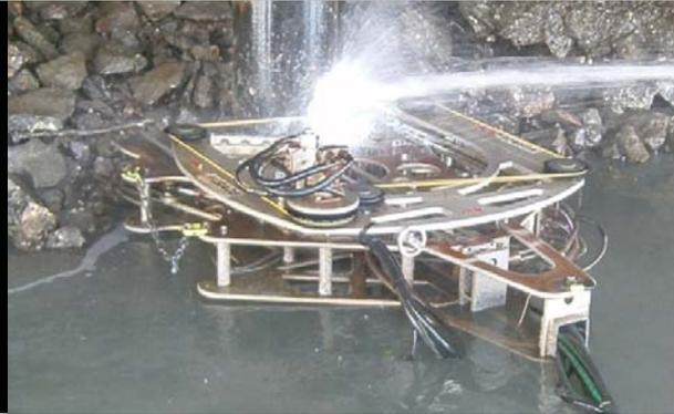
The Diamond Wire Saw cutting through a pile.
