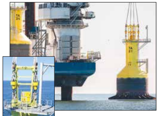
▼ Offshore wind turbine base foundations installed with a wireless SHAS-SyncHoist System to ensure the foundation remained vertical during lowering and positioning.
