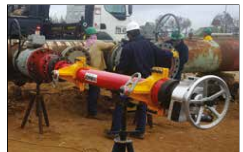
▲ CHT3000 hot tapping application for petrochemical pipeline installation.
