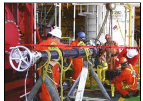
▼ CHT2000 hot tapping offshore application.
