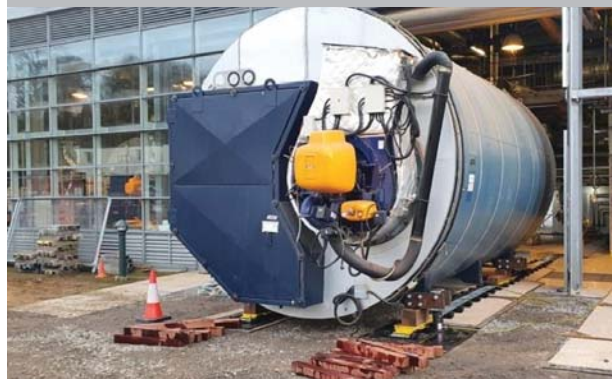
Boilers skidding in process.
