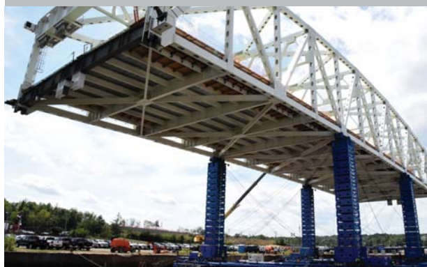
Fully lifted bridge ready for transport.
