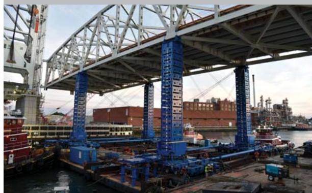
Positioning new bridge span into place.
