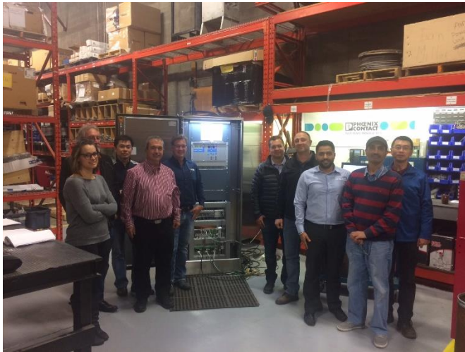
Figure 1: This project increased the expandability of the customer's system, allowing expansion and greater AMS communication.
