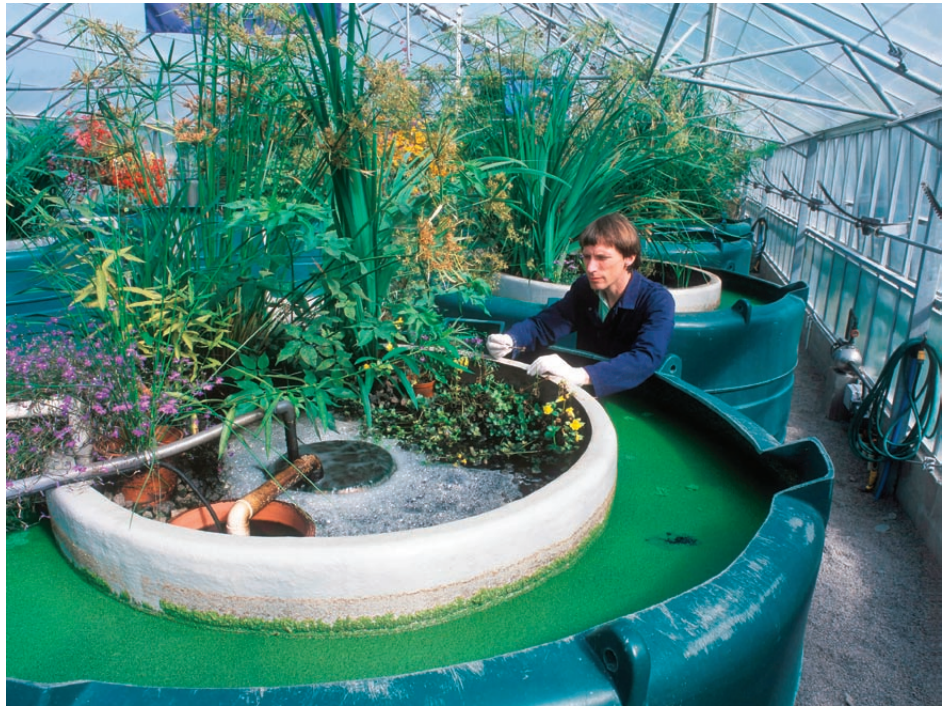
IN THE SCOTTISH ECOVILLAGE FINDHORN, THE COMMUNITY’S WASTEWATER IS PURIFIED THROUGH A TREATMENT PROCESS THAT INVOLVES VARIOUS TANKS.
